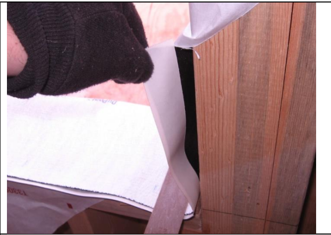
Inner strip of FlexWrap release paper makes it easy to fold up inner edge after unit is set.
